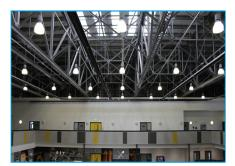
To further reduce installation times Eyre Building Services Group Ltd installed the lighting with the Gripple Express Hanger. The ergonomic buttons allow for rapid adjustment, no Setting Key required. The Express Hanger is a safer alternative to rod and channel as no tools or "Hot Works" permit is required for installation, improving health and safety on-site. The products selected complement the open soffit design of the building.
