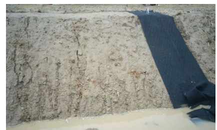
During installation of Gripple solution
