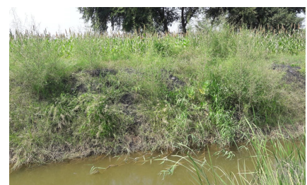
80 days after installation
