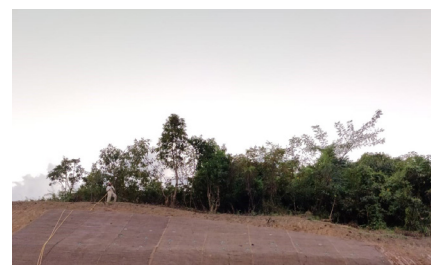
During the installation of Gripple solution
