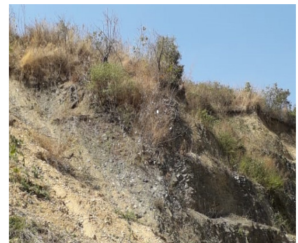
Before construction with the Gripple install
