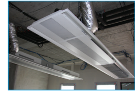
Chilled beams
