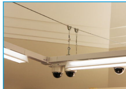
Lighting and Camera on Catenary
