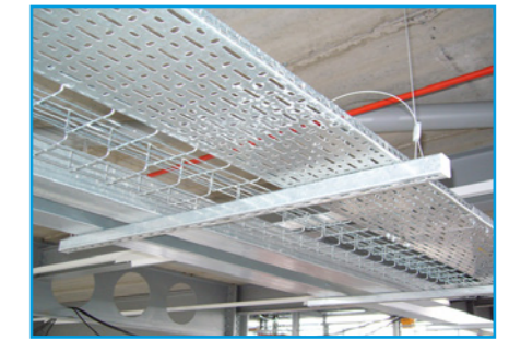
Multiple cable trays on single channel
