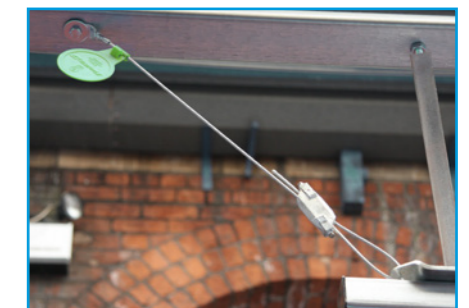
Transverse Bracing
