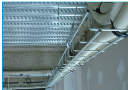
Refrigerant pipes
