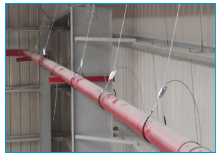
Intermediary supports for steel pipes
