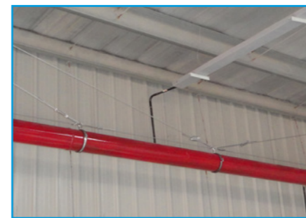
Bracing for steel pipes
