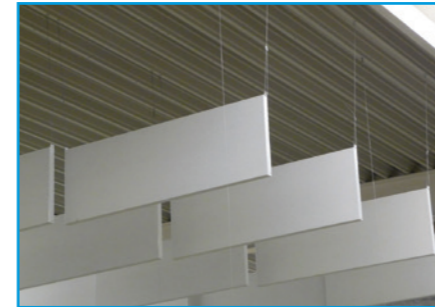
Acoustic baffles
