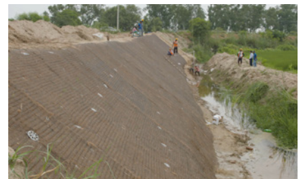
During the installation of Gripple solution
