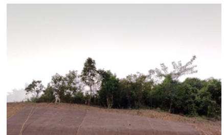
During the installation of Gripple solution
