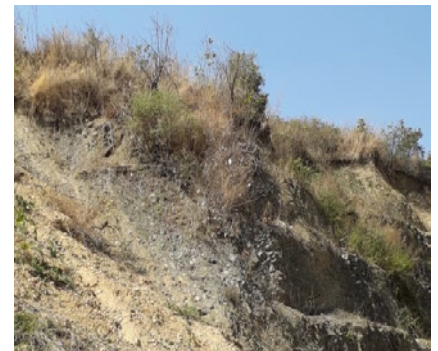
Before construction with the Gripple install
