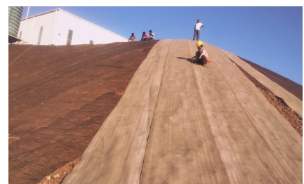
Concrete Canvas installed with the Gripple Terra-Lock™ System
